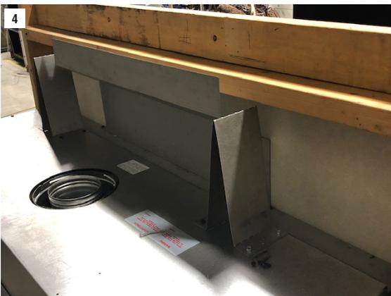
3. Finish out wall with 1/2" finishing materials – paint with high-temperature paint, etc.
