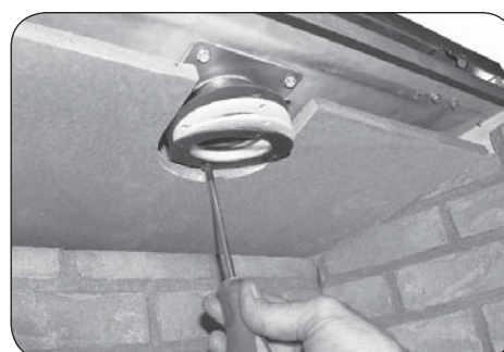
Fig. 54-4 Install plate and gaskets
