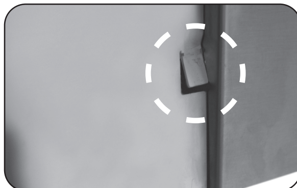
Fig. 24-4 Tab slightly bent in for clearance
